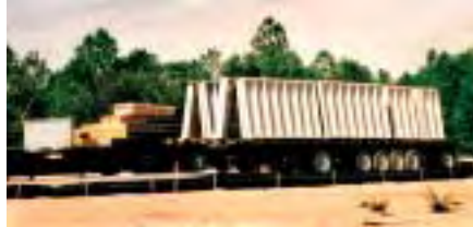
Photograph 10 Pre-cast basement walls
