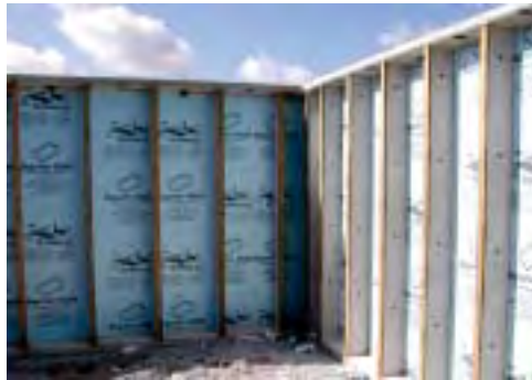
Photograph 11 Pre-cast basement walls with XPS foam insulation
