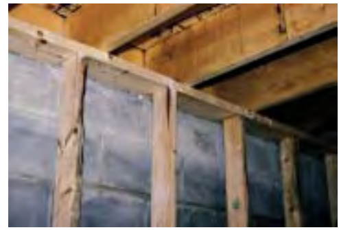
Photograph 1 Interior stud framing located at basement perimeter
